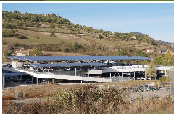
Ombrière de parking, Creissels (12). © Étienne Louyriac
