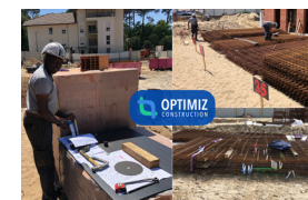
Photos : Optimiz Construction
