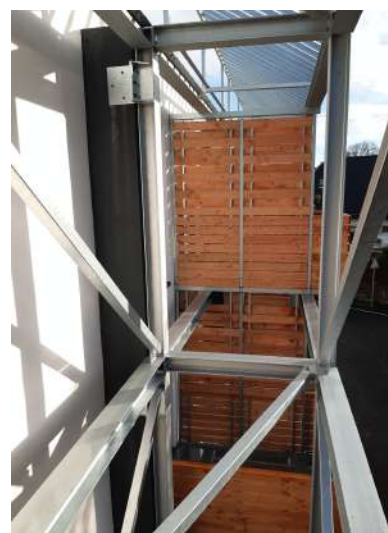
Façade sud Photos © RBBD
